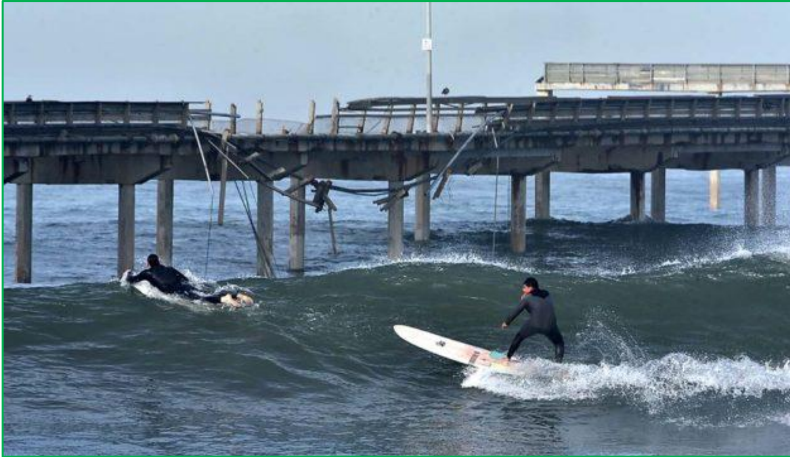
A surfer passes the damage to the railing of the Ocean Beach Pier during the king tide, peaking about 8 a.m. Jan 18 with an expected 7.3 tide. Photo by Chris Stone
