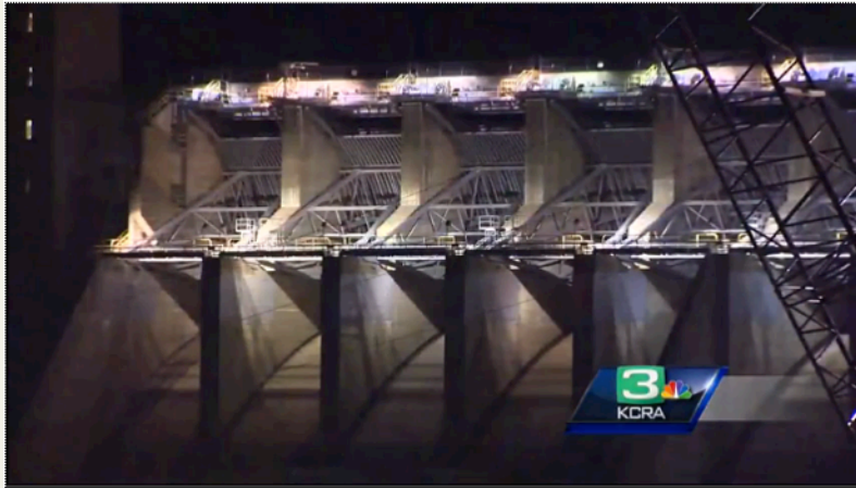
Feb. 9: Folsom, CA. Reservoir operators are nearly doubling the amount of water outflow from Folsom dam to make room for the above average Sierra snowpack and future storms.
