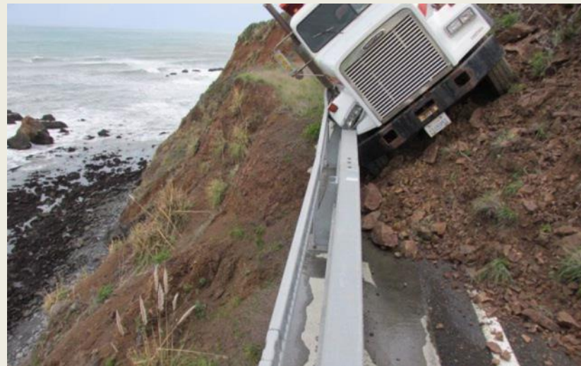
March 11: A Caltrans employee and his dump truck were hit by a mudslide on Highway 1 in Mendocino while responding to an earlier mudslide. Photo, SF Gate
