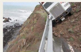
March 11: A Caltrans employee and his dump truck were hit by a mudslide on Highway 1 in Mendocino while responding to a earlier mudslide. Photo: SF Gate
